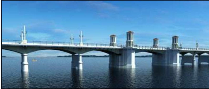
Photo 5-68. View of the Rehabilitated Bridge of Lions
