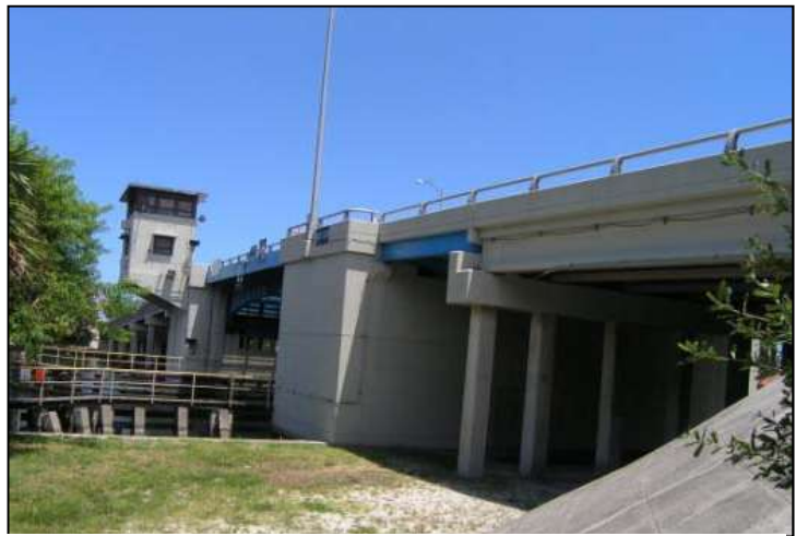
Photo 5-69. Davie Boulevard Bridge, Broward County (No. 860038)
