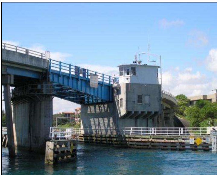
Photo 5-72. Boca Inlet Bridge, Palm Beach County (No. 930060)
