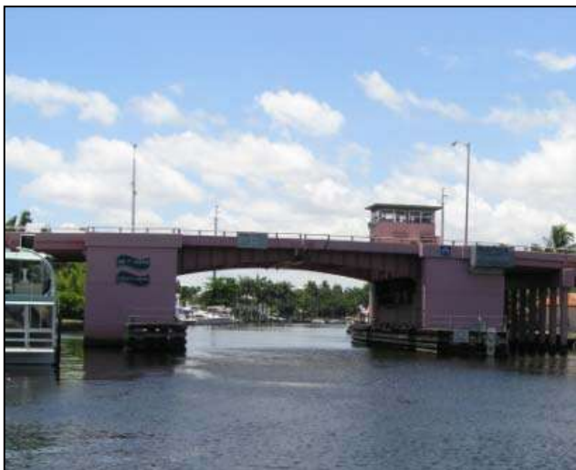
Photo 5-70. William H. Marshall Memorial Bridge, Broward County (No. 864072)
