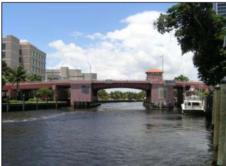
Photo 5-71. SE 3 rd Avenue Bridge, Broward County (No. 864071)
