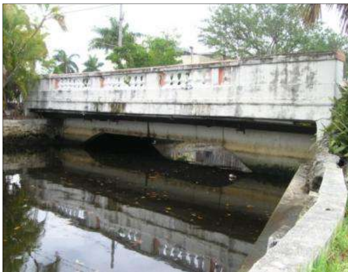
Photo 5-12. Grand Canal Arch Deck Bridge, Broward County (No. 865732)
