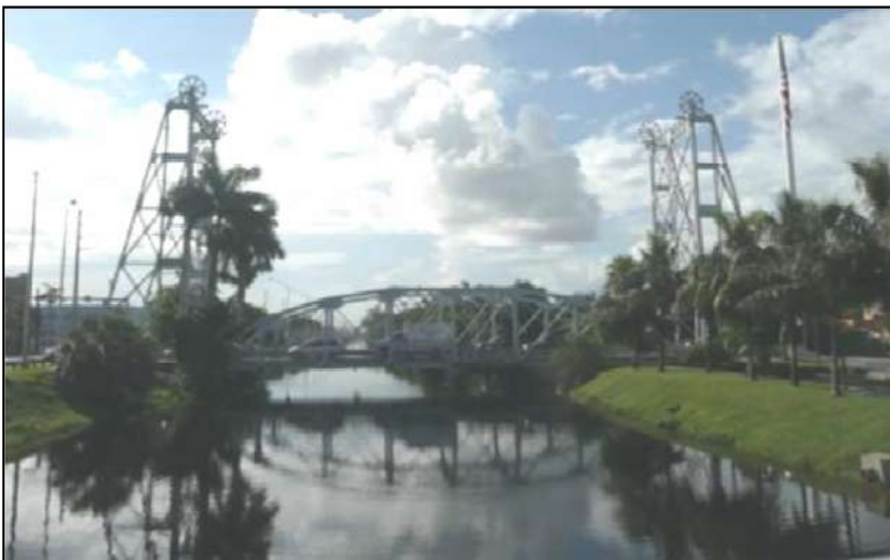
Photo 5-54. Hialeah-Miami Springs Vertical Lift Bridge, Miami-Dade County (No. 874129)
