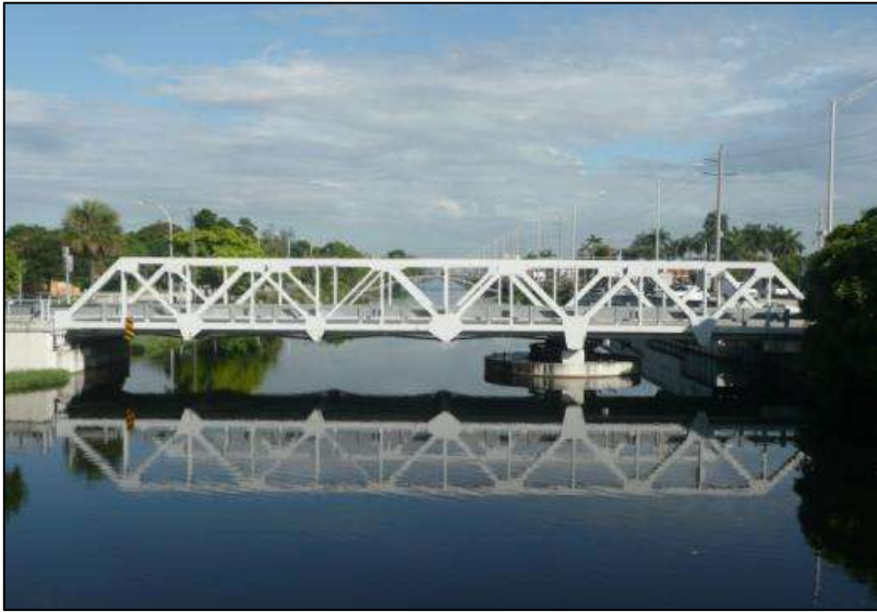
Photo 5-62. Miami River Canal Swing Bridge, Miami-Dade County (No. 874130)
