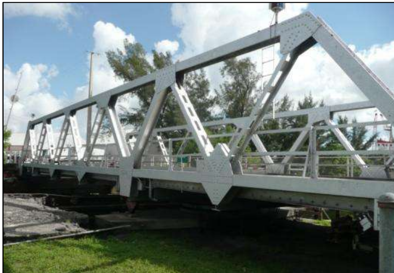
Photo 5-63. Tamiami Canal/NW South River Dr. Swing Bridge, Miami-Dade County (No. 874135)
