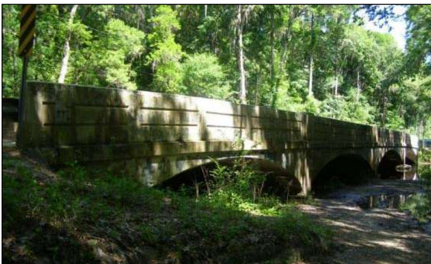
Photo 5-17. North Crystal Springs Bridge, Pasco County (No. 144002)
