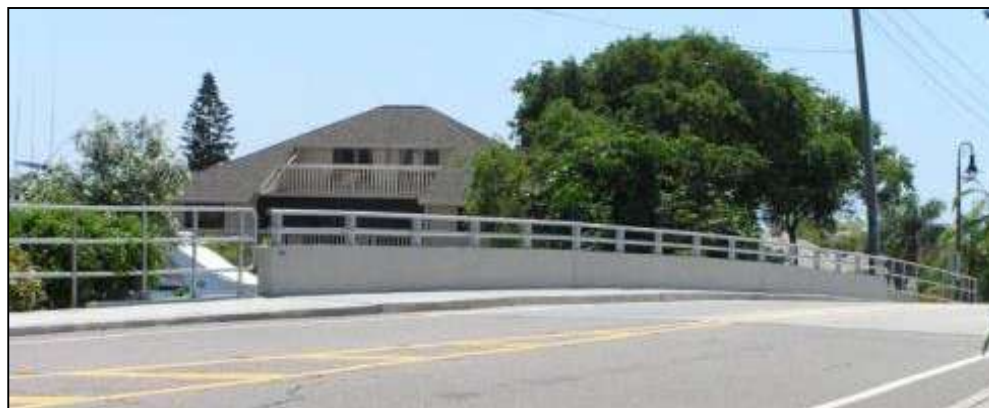
Photo 7-13. Madonna Boulevard Bridge with Replaced Railing, June 2010.
