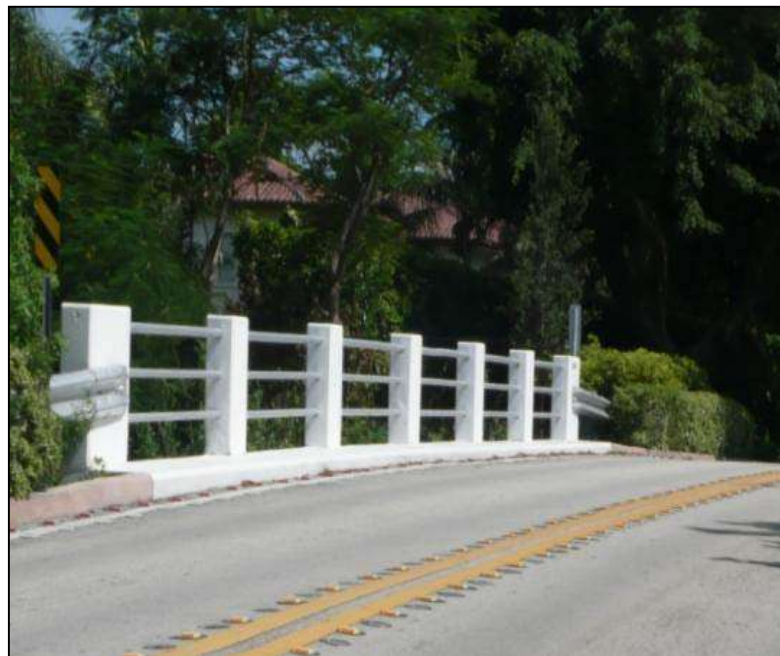
Photo 7-15. The Granada Boulevard Bridge with Replaced Railing, 2010.
