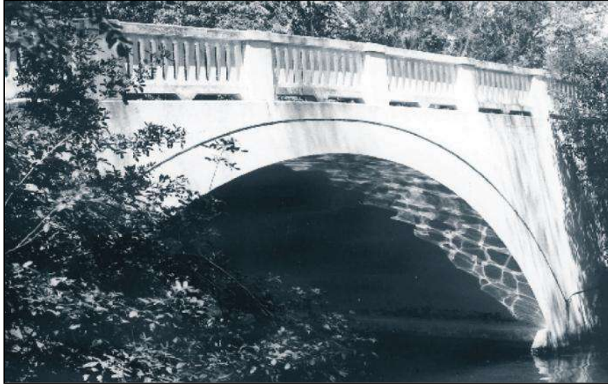
Photo 7-14. Original Appearance of the Granada Boulevard Bridge.
