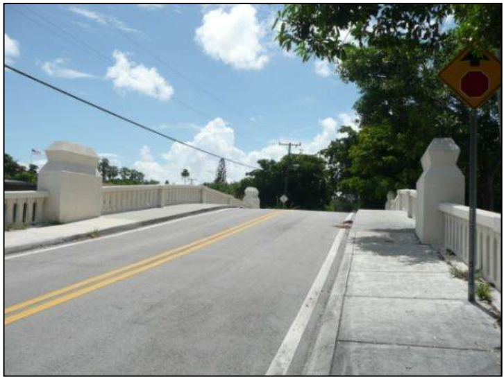
Photo 5-15. Seybold Canal Bridge, Miami-Dade County (No. 876500)
