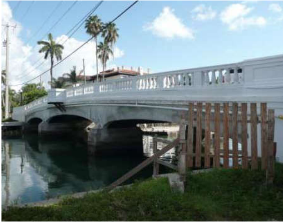
Photo 6-7. Sunset Island Bridge No. 1 (No. 876707)
