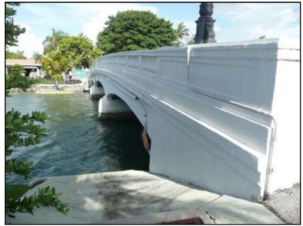
Photo 6-8. Sunset Island Bridge No. 4 (No. 876710)
