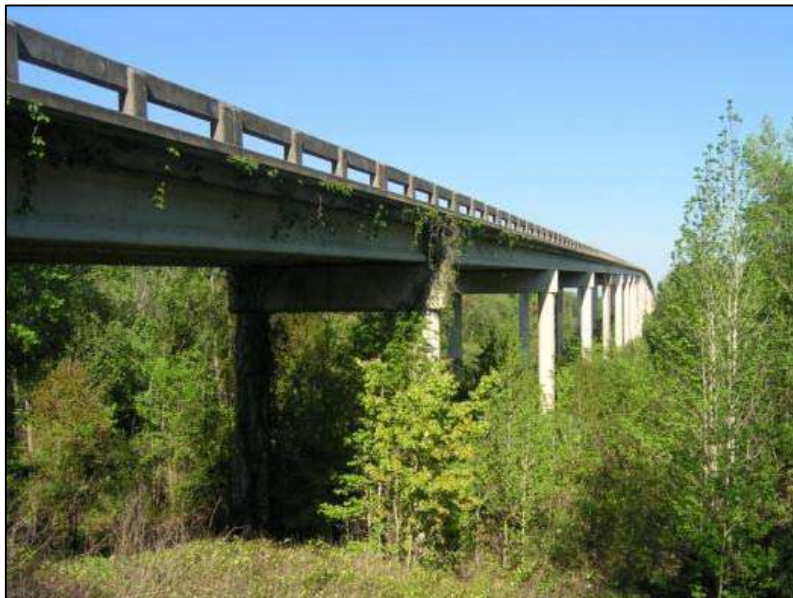
Photo 5-43. CR-316 over Proposed Cross Florida Canal, Marion County (No. 364040)
