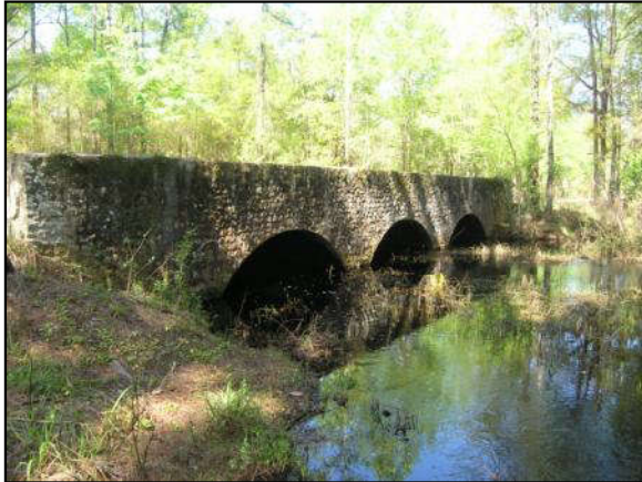
Photo 6-19. SE 137 th Avenue Creek Culvert, Marion County (No. 364120)
