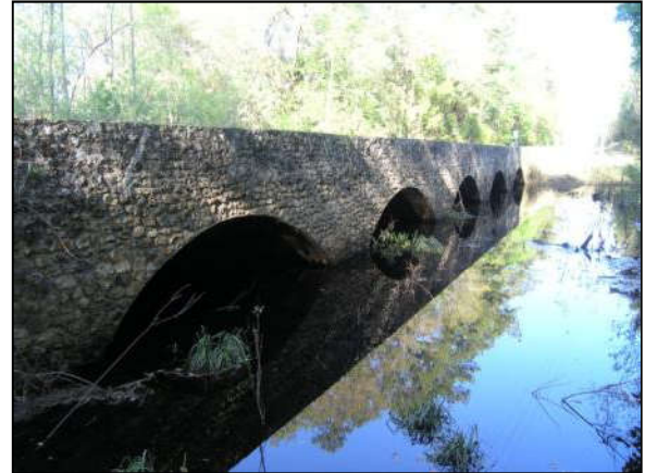
Photo 6-20. NE 105 th Street Culvert over Daisy Creek, Marion County (No. 364060)
