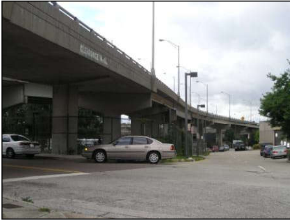
Photo 6-29. SR-228 at Adams Street Prestressed Concrete Bridge (No. 720496)
