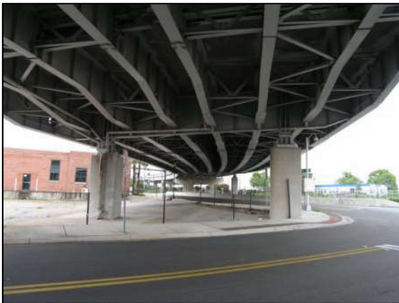
Photo 6-31. SR-228 (Leg G) Bridge (No. 720490)
