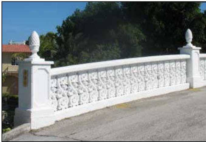
Photo 6-5. Harbour Bridge (No. 904604)
