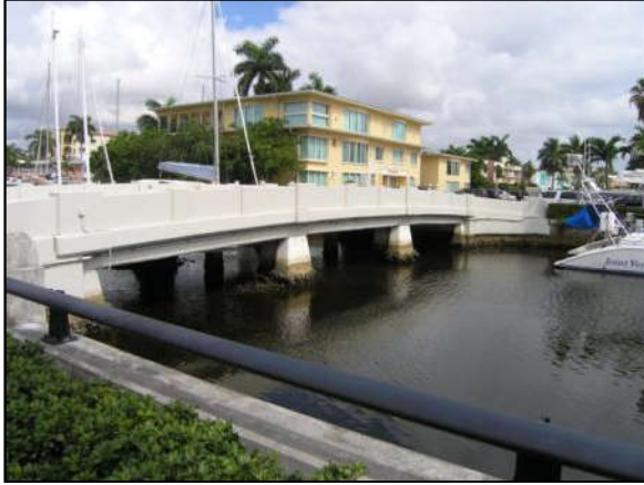
Photo 6-1. Isle of Venice Bridge (No. 865734)
