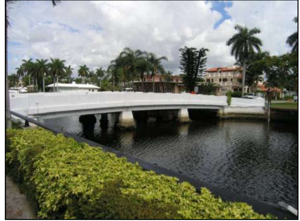
Photo 6-2. Royal Palm Drive Bridge (No. 865737)
