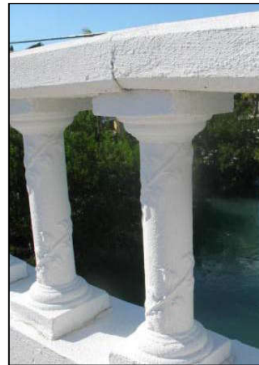
Photo 6-6. Rosen Bridge (No. 904606)
