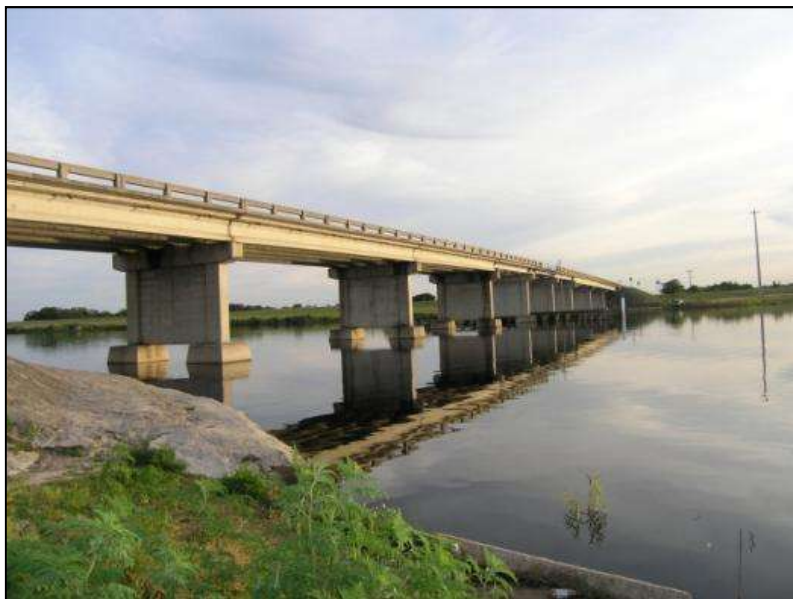
Photo 5-38. SR-78 Bridge, Okeechobee County (No. 910009)
