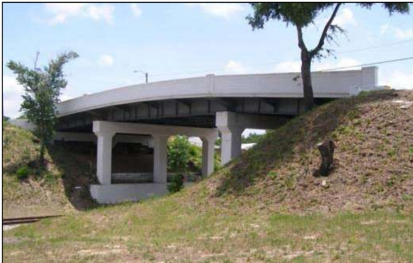
Photo 5-37. Haines City Overpass, Polk County (No. 165700)
