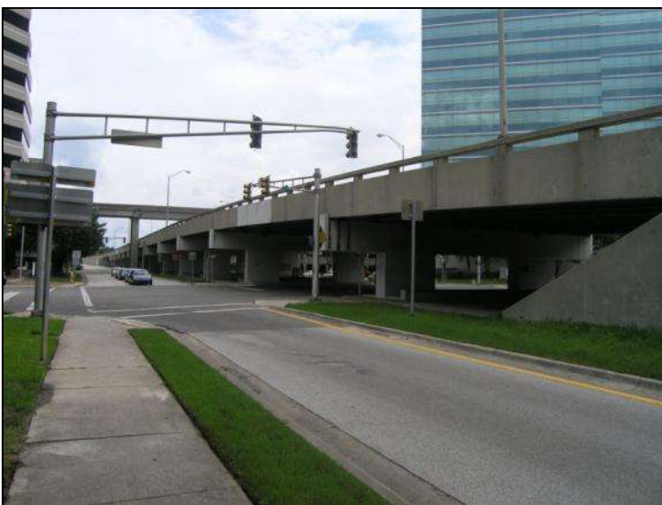
Photo 5-40. US-1/SR-5 Bridge over Miami Road, Looking Southwest, Duval County (No. 720087)
