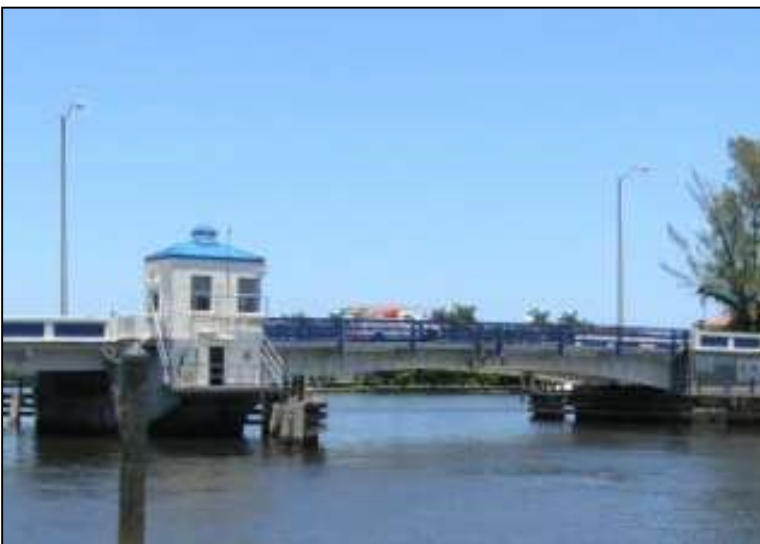
Photo 5-73. George Bush Boulevard Bridge/NE 8 th Street Bridge, Palm Beach County (No. 930026)
