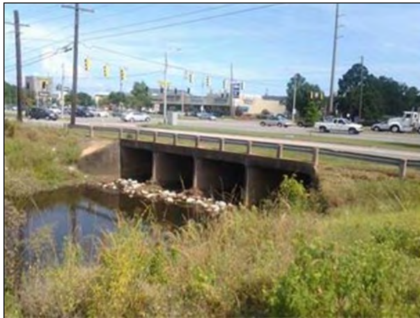
Figure 8.4. Airport Boulevard over Montlimar Creek from upstream.
